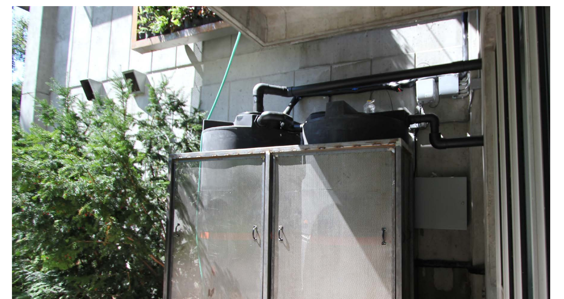
Two 1,000 cisterns recycle roof water for irrigation. Average daily water use (~5 gal) as well as amount of potable back up water (0 gal since Sept 2014) are being documented.
