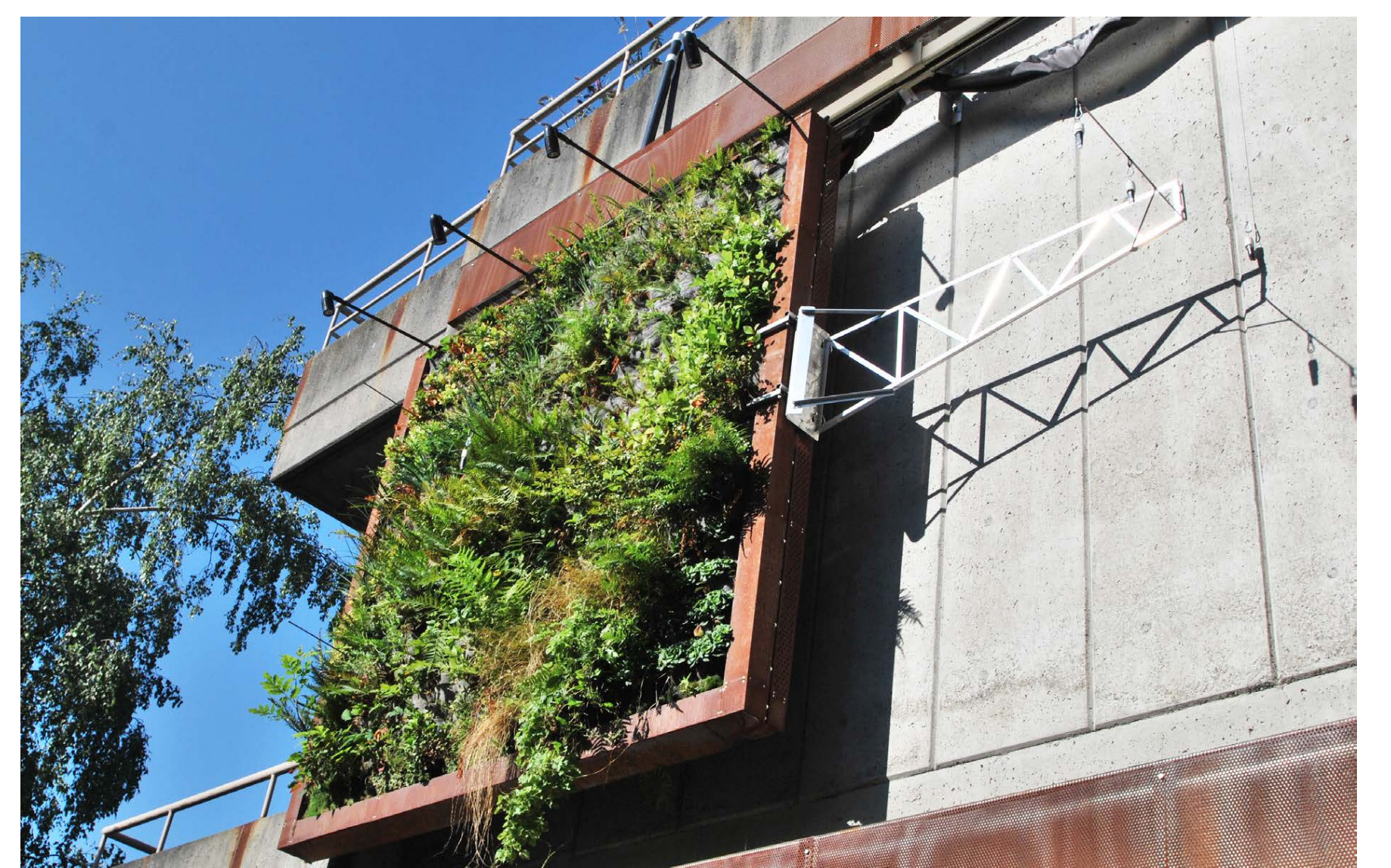
Temperature sensors measure how the green wall is affecting the urban heat island effect (~3° C) and building performance (~0.5° C).
