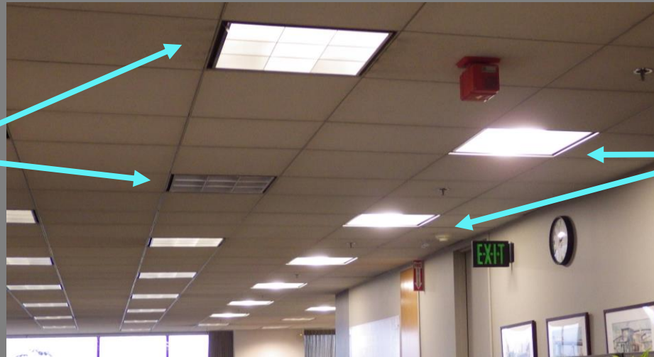
December 2015, 12 th Floor of UW Tower
