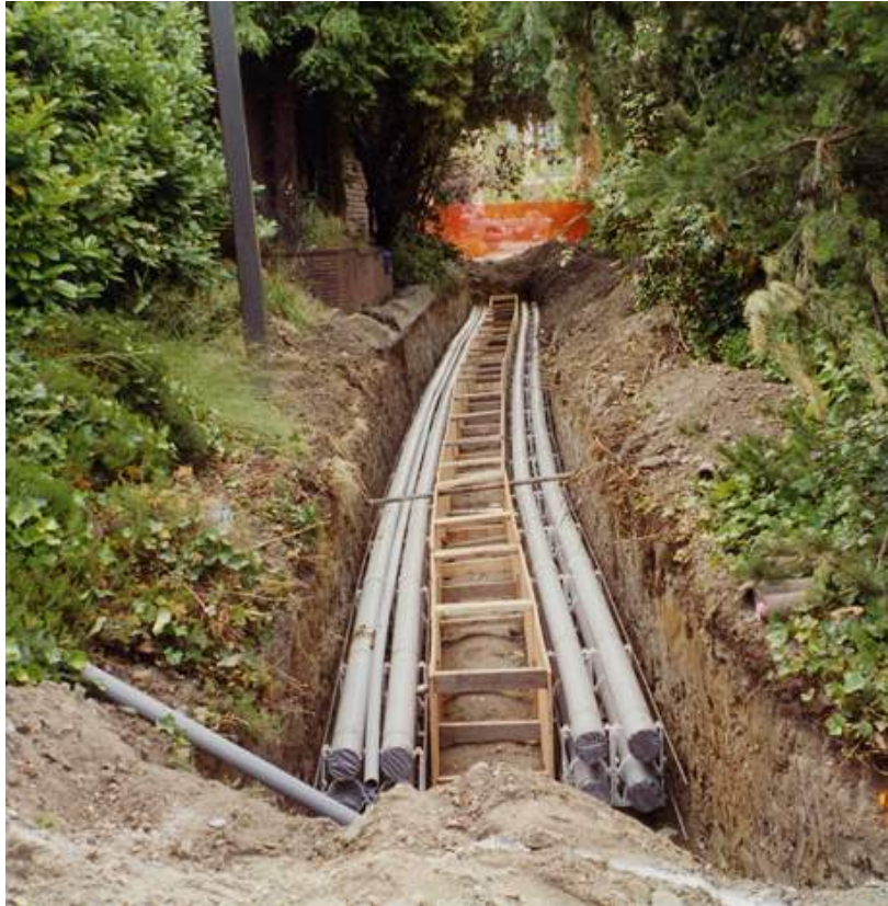
Figure 4.3.1-2: Photo of a previous electrical duct bank installation through Burke Gilman Trail
