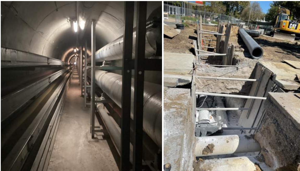
Figure 4.3.1-1: Photo of an existing campus utility tunnel (left) and an in-progress shot of direct-bury piping installation from another campus (right)
