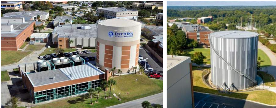
Figure 4.2.2.1-10: Thermal Energy Storage tanks at Daytona State (left) and North Carolina State Raleigh (right)
