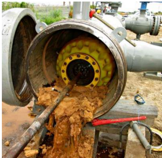
Figure 3-27. Pipeline pigging, courtesy of Enduro Pipeline Services
