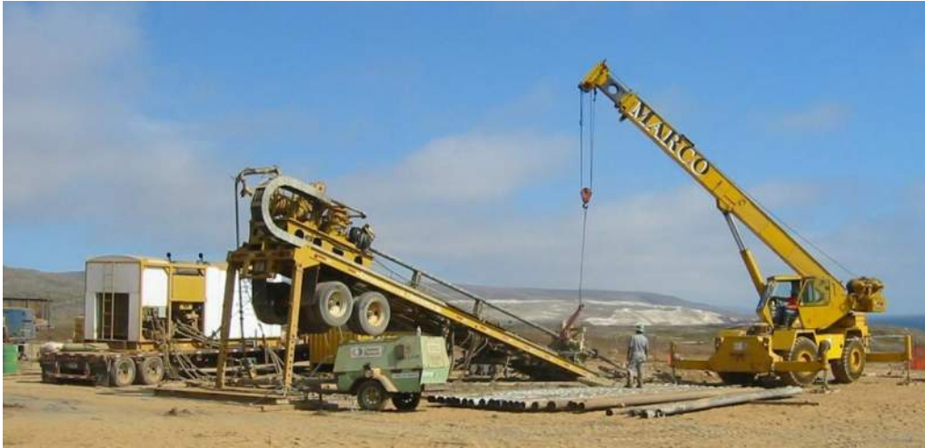
Figure 3-30. HDD drill rig, pipe, and support equipment on land.
