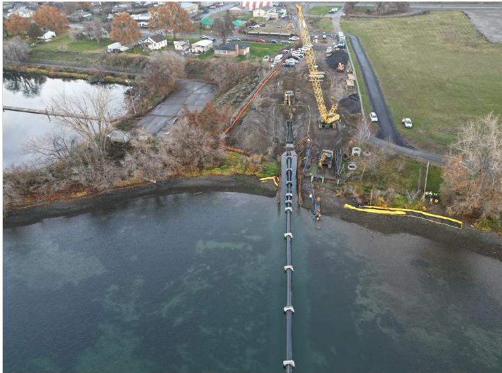
Figure 3-42. Installation of City of Pasco outfall pipeline in the Columbia River, courtesy of Advanced American Construction.
