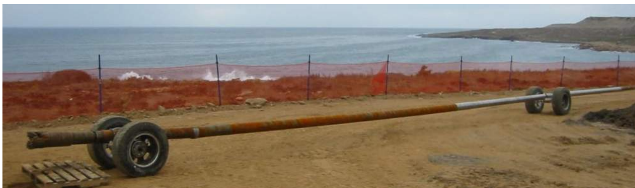
Figure 3-32. HDD DHA on temporary wheels.
