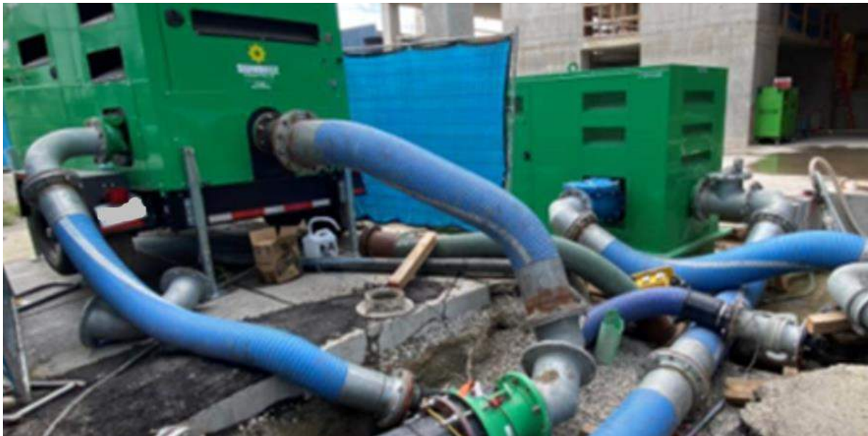
Figure 1.2.1 Temporary bypass pumping trailers.
