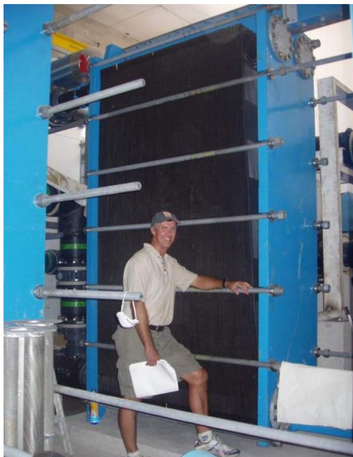
Figure 3-18. Photo of a Makai engineer next to a 0.8 MW plate frame heat exchanger (PFHE). The UW LSCH project is 22.3 MW for comparison, requiring a series of PFHEs.
