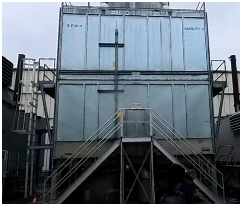
Figure 1.1.2 Photo from cooling tower arrangement with elevated support structure and access platforms.
