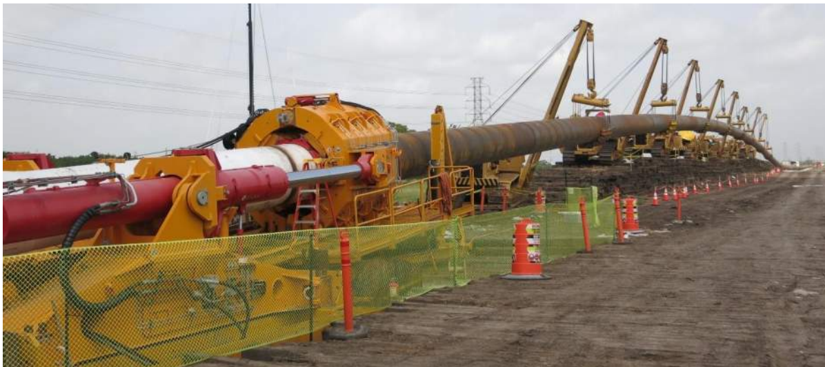
Figure 3-38. Photo of a low angle Direct Pipe launch showing the pipe thruster and pre-assembled steel casing pipe on land, courtesy Michels.
