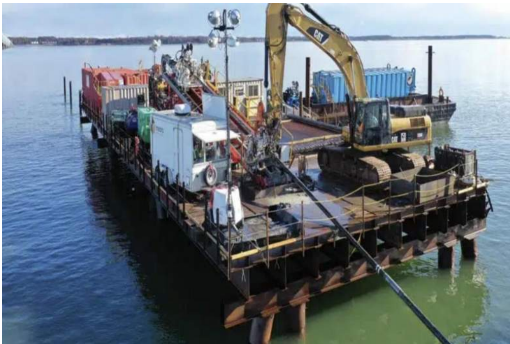
Figure 3-31. HDD drill rig, pipe, and support equipment on a barge.
