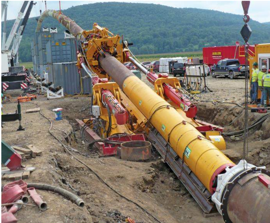
Figure 3-37. Photo of a high angle Direct Pipe launch showing the microtunnelling machine (yellow) and pipe thruster (red and yellow).
