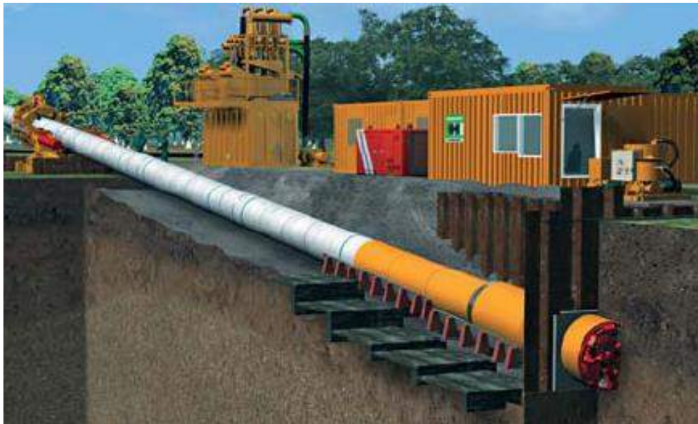
Figure 3-36. Microtunneling machine starting a borehole, courtesy Herrenknecht.
