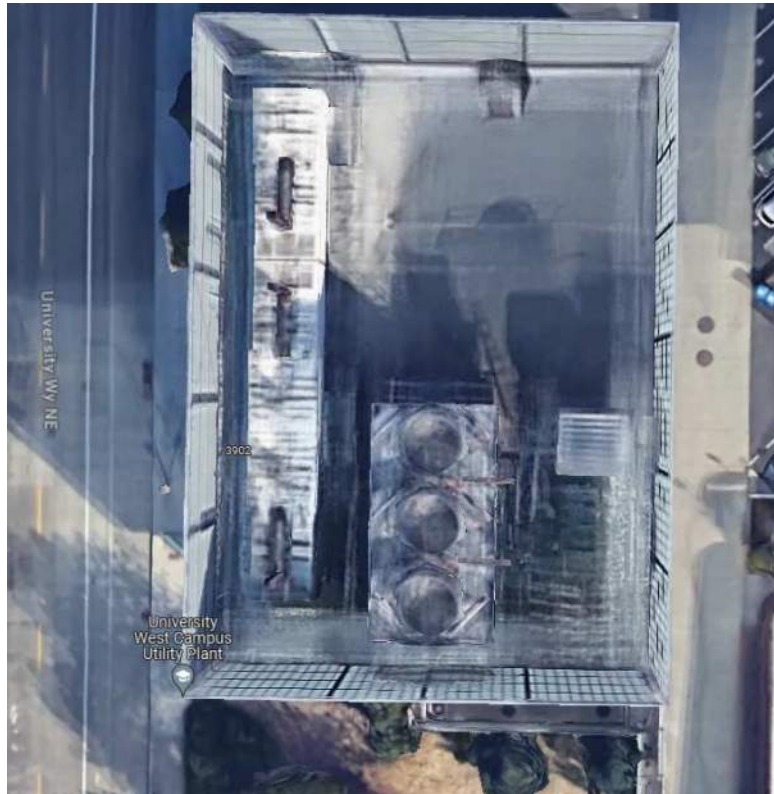
Figure 1.1.3 Satellite image of existing WCUP roof condition. WCT5 will be installed adjacent to the existing cooling tower array.
