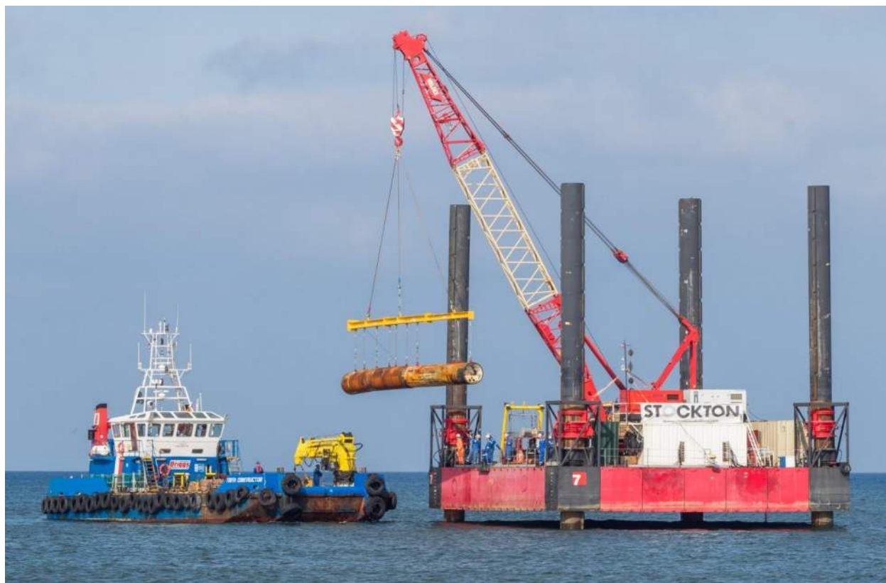
Figure 3-39. Tunneling machine in-water recovery after borehole completion, courtesy Mears.
