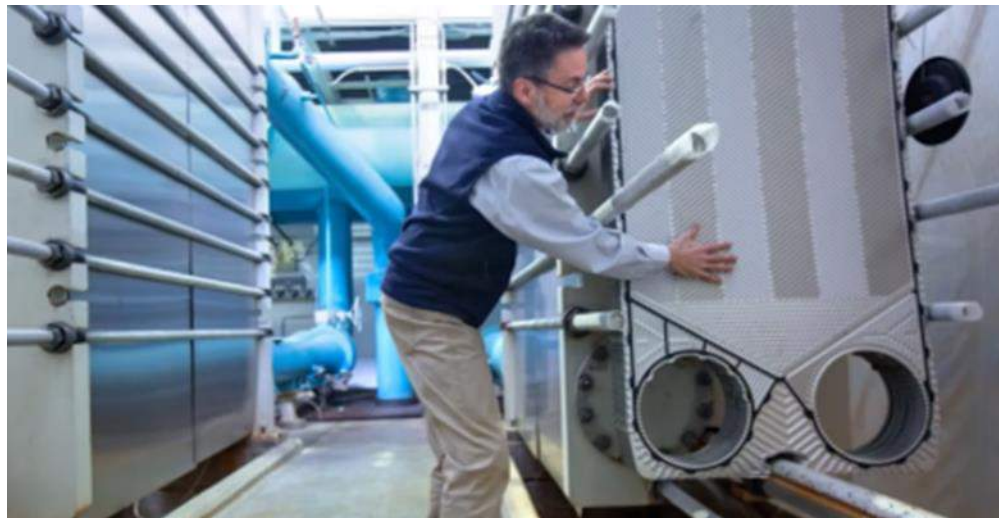
Figure 3-20. Photo of heat exchanger plate replacement inside the Lake Source Cooling facility, courtesy of Cornell University
