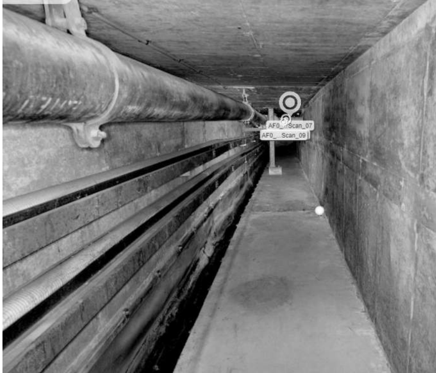
Figure 3.4.5-3: Tunnel section between AF 0 and AF 1. Domestic water piping routed high, electrical distribution racked along left wall, and drainage trench on bottom left.
