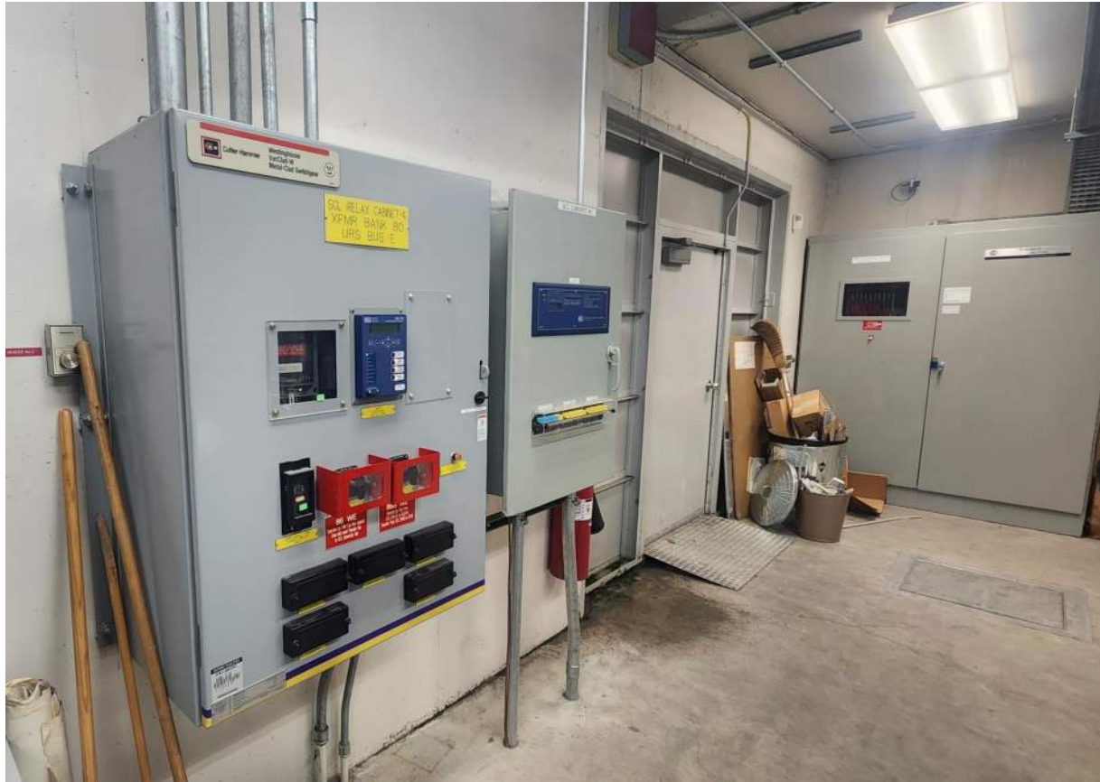
Figure 3.4.2-3: WRS overcurrent protection SEL relays and SCL primary metering.
