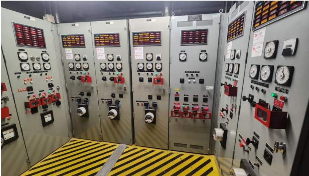
Figure 3.4.3-4: Emergency and standby generator paralleling gear at the Power Plant.
