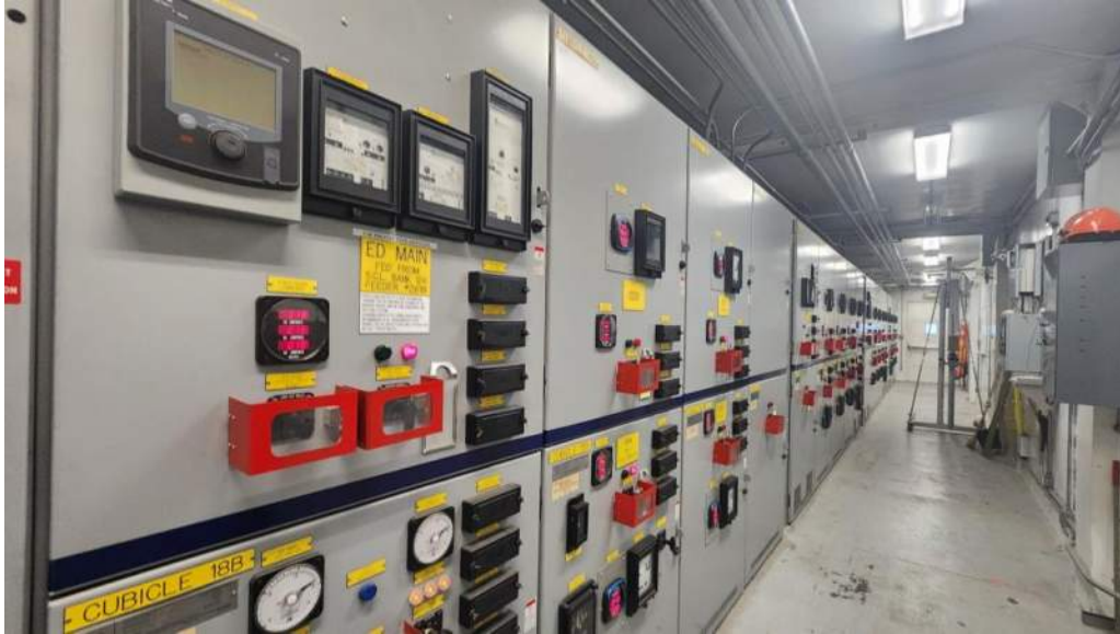
Figure 3.4.4-2: ED Main where the SCL service enters the ERS.
