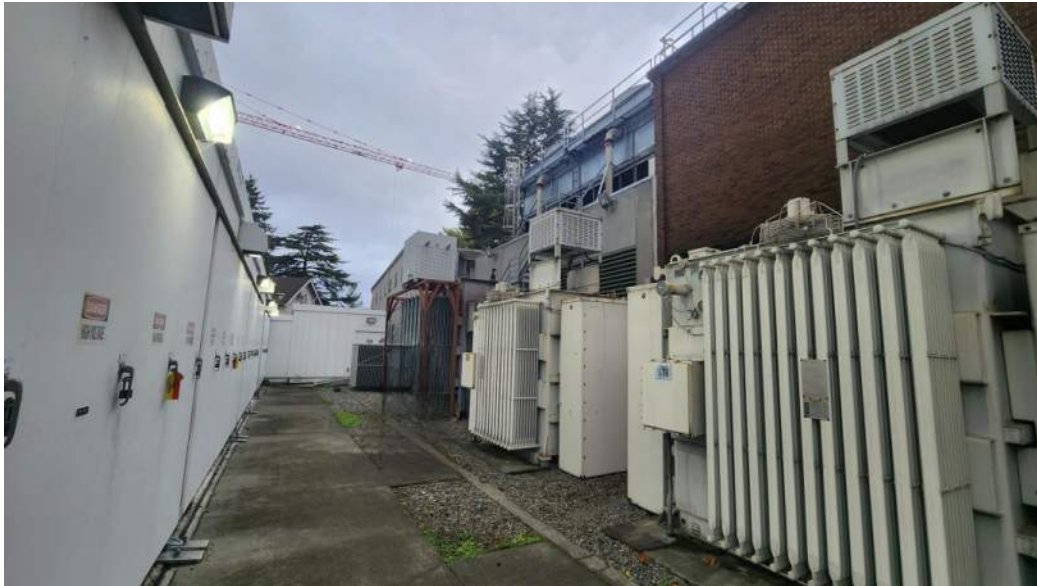
Figure 3.4.4-1: East Receiving Station (ERS) transformer yard and switchgear.
