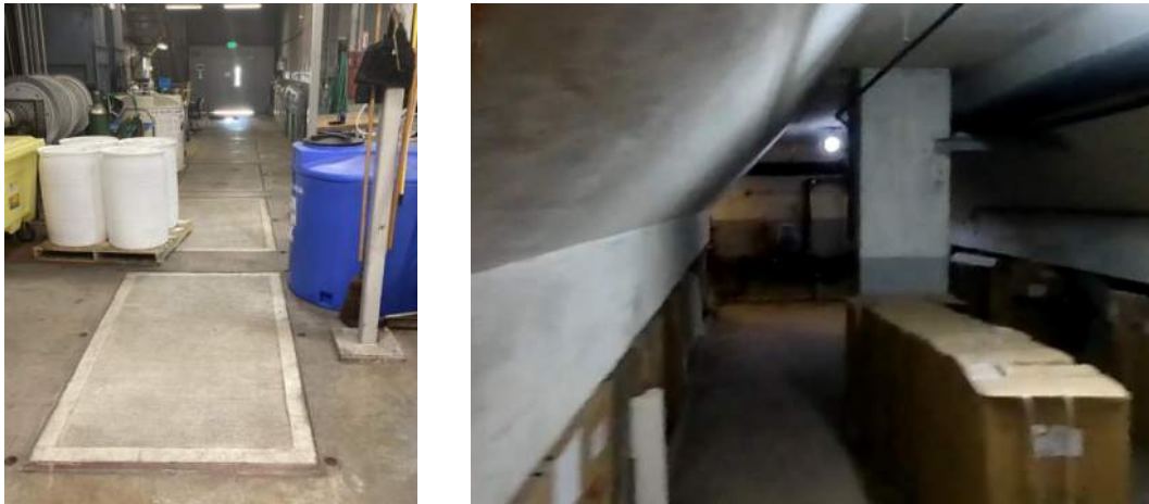
Figure 3.4.3-2: Top (left) and bottom (right) of coal bunkers in basement area of plant. Nearly 20-30 feet of height within the tanks (to be confirmed).
