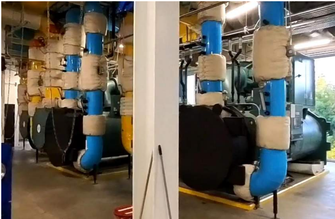
Figure 3.4.1-1: WCUP water-cooled chillers 1 through 3.
