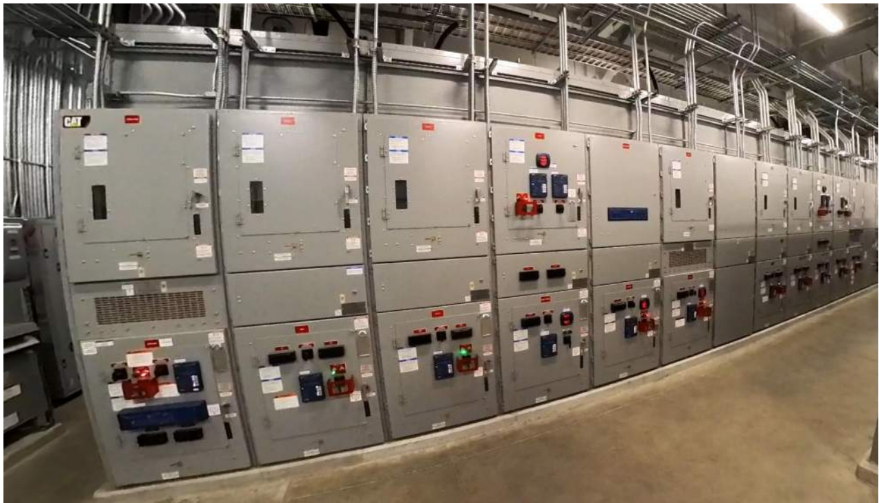
Figure 3.4.1-5: WCUP 4160V switchgear in main electrical room.
