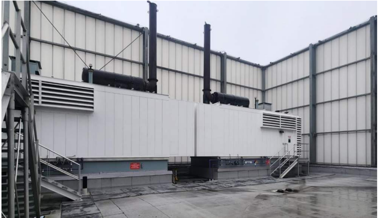
Figure 3.4.1-4: WCUP Diesel generators on the roof. Two of the four pictured.
