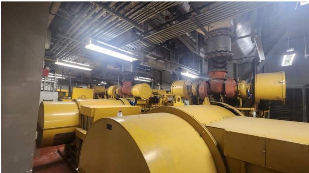
Figure 3.4.3-5: Diesel generator room.
