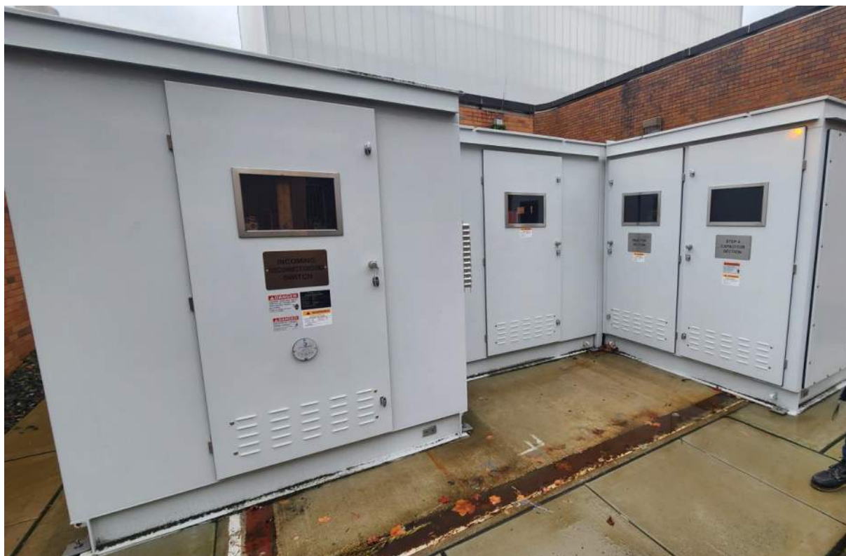
Figure 3.4.2-2: Capacitor bank at WRS.
