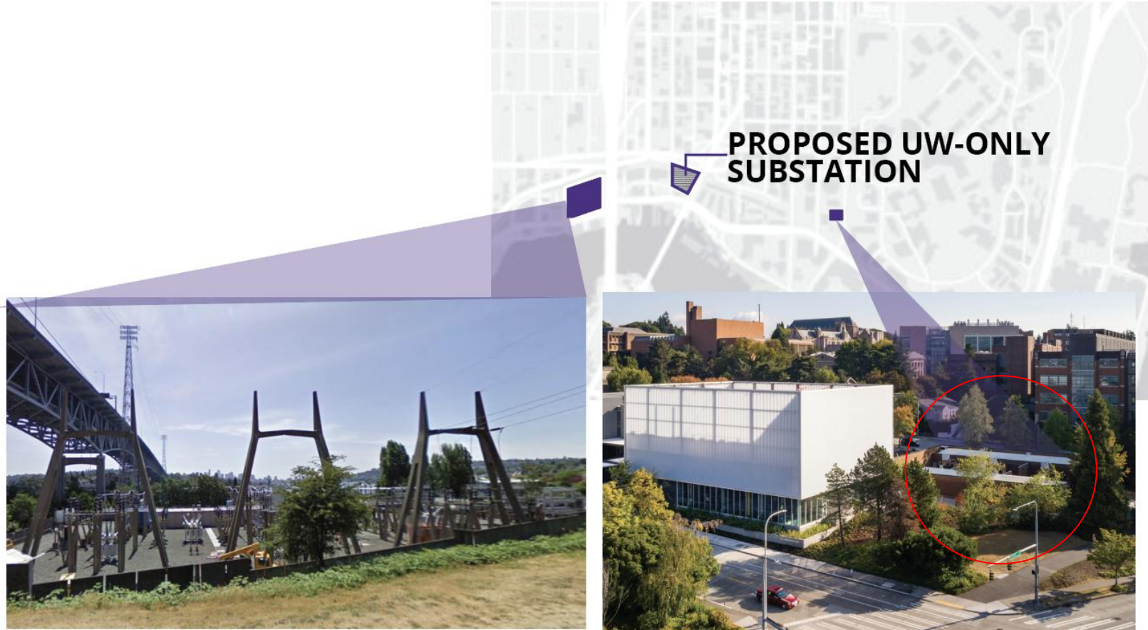
UNIVERSITY DISTRICT SUBSTATION
