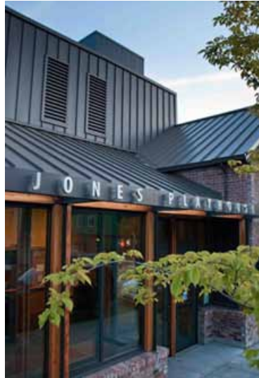
Lobby Operable Windows
