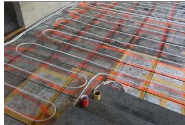
Under Floor Heating System Being Installed
