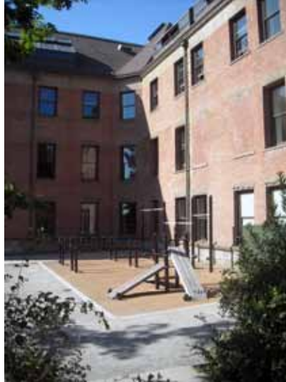
N.E. Corner of Clark Hall Fitness Area
